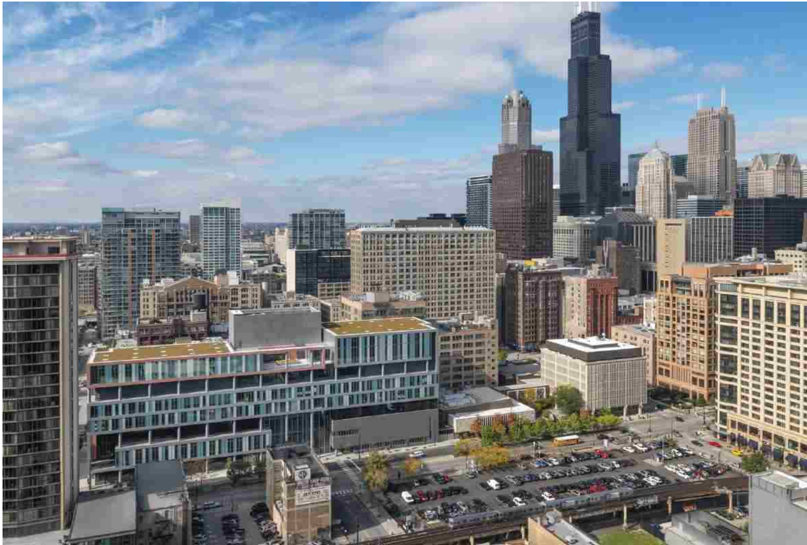
Figure 15 - William Jones Preparatory School with Context
